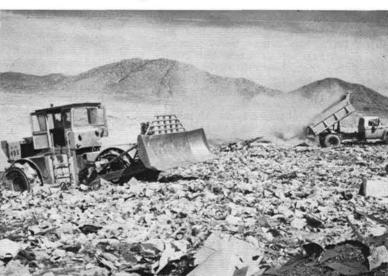
THE CRUNCHER, or whatever this machine is called, weighs some 35 tons and is used to break down and compact trash, after which a dozer pushes trash plus earth into the big hole previously excavated by the dozer. When hole is filled after 2-3 months, operation moves on to new site.
